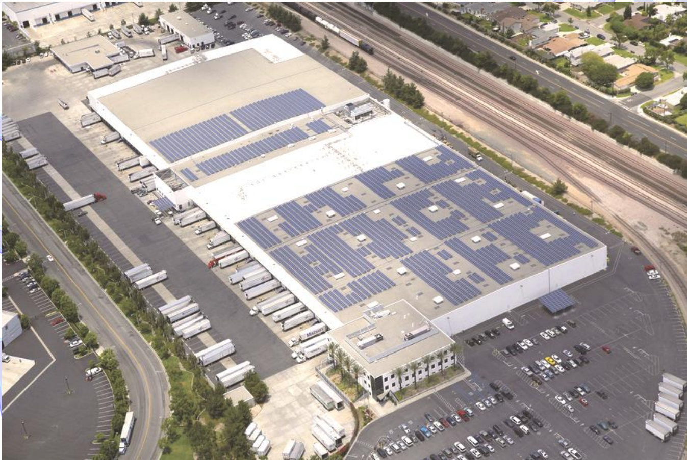
Solar park at the U.S. Foods' facility in La Mirada, California
